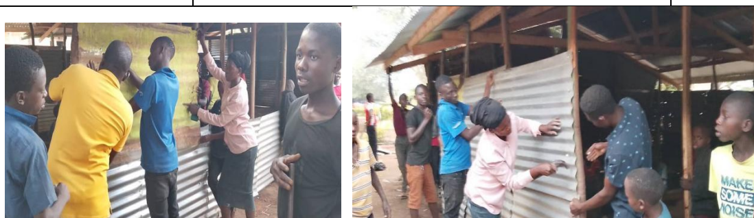
Figure 51 Intern Participated in the construction of two classrooms using iron sheets with school director, teacher, workers and pupils
