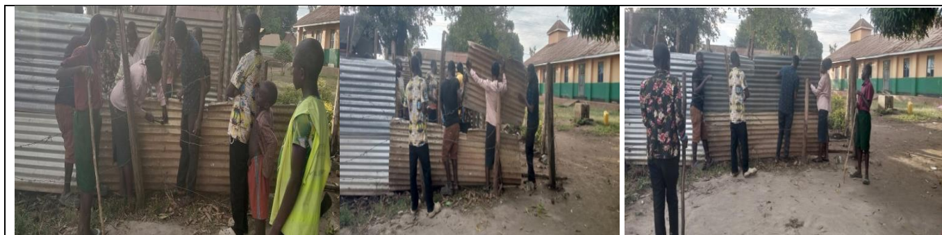
Figure 52: The intern participated in the construction of one bathroom for boys
