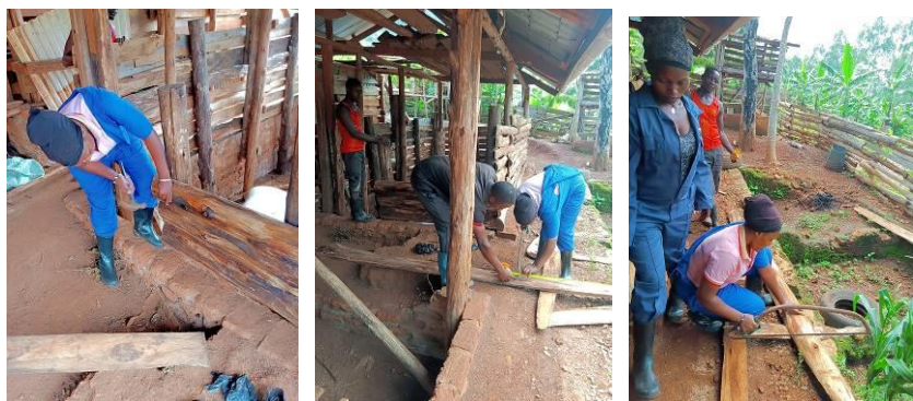
FIGURE 1,2, AND 3 WE WERE ATTACHING POLES ONTO THE POSTS ON LENGTH
