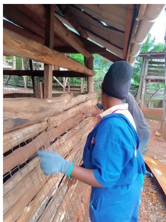
FIGURE 2 INSTALLING WIRE MESH
