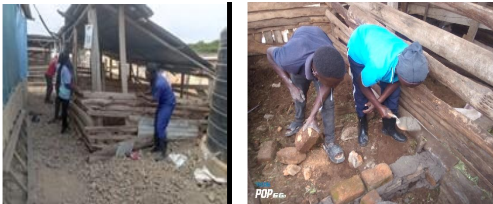
Figure 10. The apprentice nailing wood into a broken pig sty and laying bricks on a broken feed trough.
