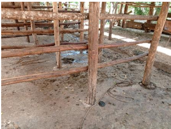
Figure III 32:Before cleaning the kraal
