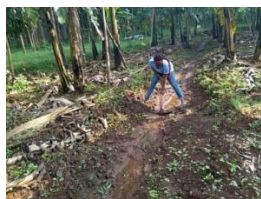
Figure 30. Digging of trenches
