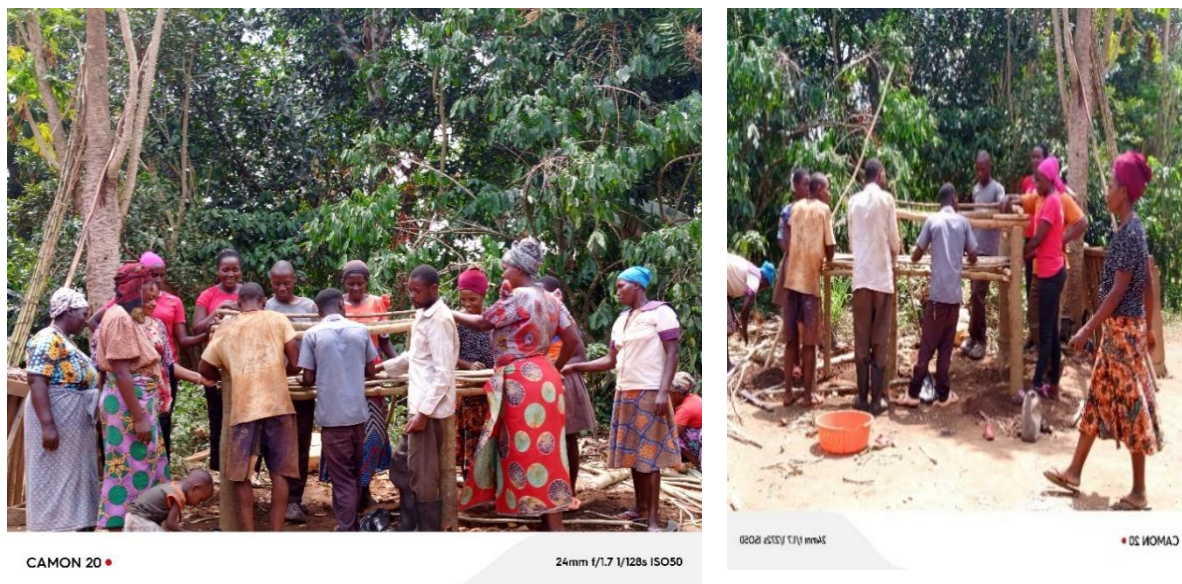
Figure 11 An intern participating in the construction of drying rack
