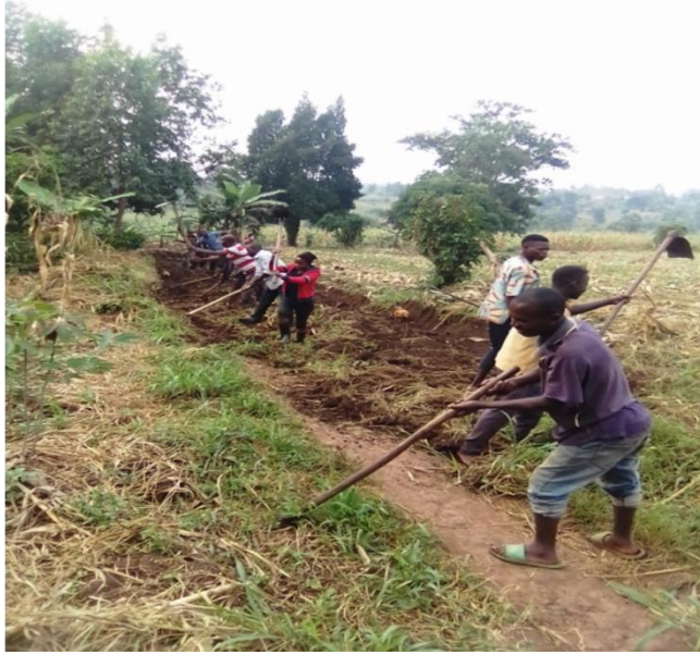
Photo 15: The Intern participating in clearing of Kasambya road with community members
