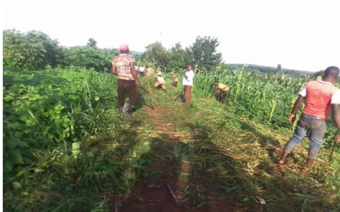
Photo 14: The community members slashing Kyamururu road together with the Intern
